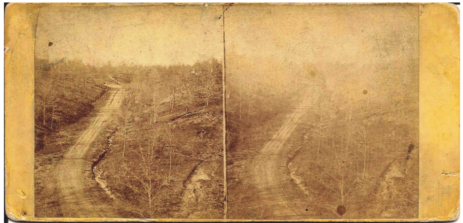
The road running west through the valley from the Oak Ridge Cemetery's Third Street entrance. It was along this road that the Lincoln funeral procession passed on the afternoon of May 4, 1865, stopping at the Receiving Vault where Lincoln's body was placed. The stereoview was taken by Ridgeway Glover of Schrieber and Glover, Philadelphia photographers. Glover was present at Lincoln's funeral and took this stereoview at the time of the funeral in early May 1865.
